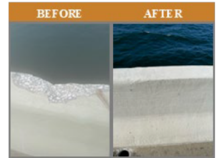
FIGURE 11. SPALL REPAIR ON SUNSHINE SKYWAY CORRIDOR IN FLORIDA
